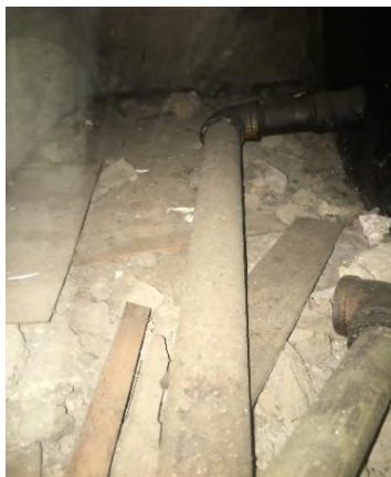
PHOTOGRAPH 11: Drain connection at tank.
