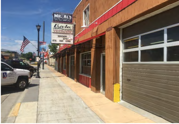
PHOTOGRAPH 31: Front of building viewing west.
