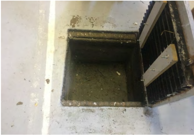
PHOTOGRAPH 1: Floor trap in northeast corner of building.
