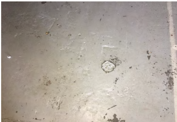
PHOTOGRAPH 21: Evidence of patches in floor above used oil storage tank.
