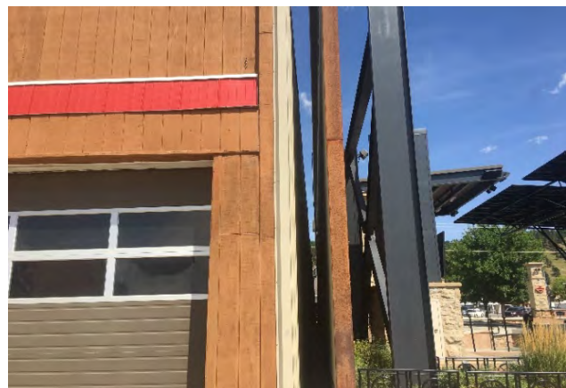
PHOTOGRAPH 30: Exterior wall along east border of property.
