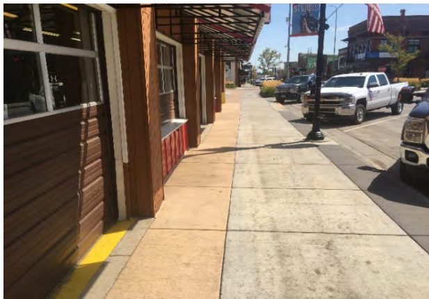
PHOTOGRAPH 29: Front sidewalk along main street looking east.
