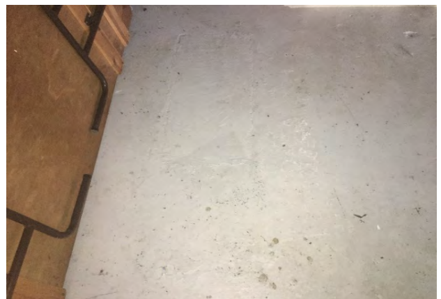
PHOTOGRAPH 22: Evidence of patches in floor above used oil storage tank.
