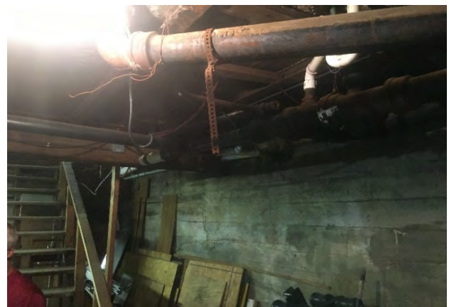
PHOTOGRAPH 6: Viewing northwest at northwest corner of basement.
