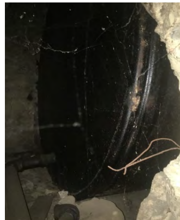
PHOTOGRAPH 12: Tank set in wall in basement.
