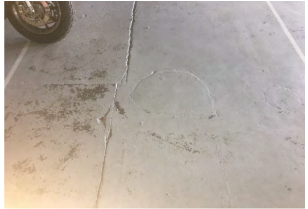
PHOTOGRAPH 20: Evidence of patches in floor above used oil storage tank.
